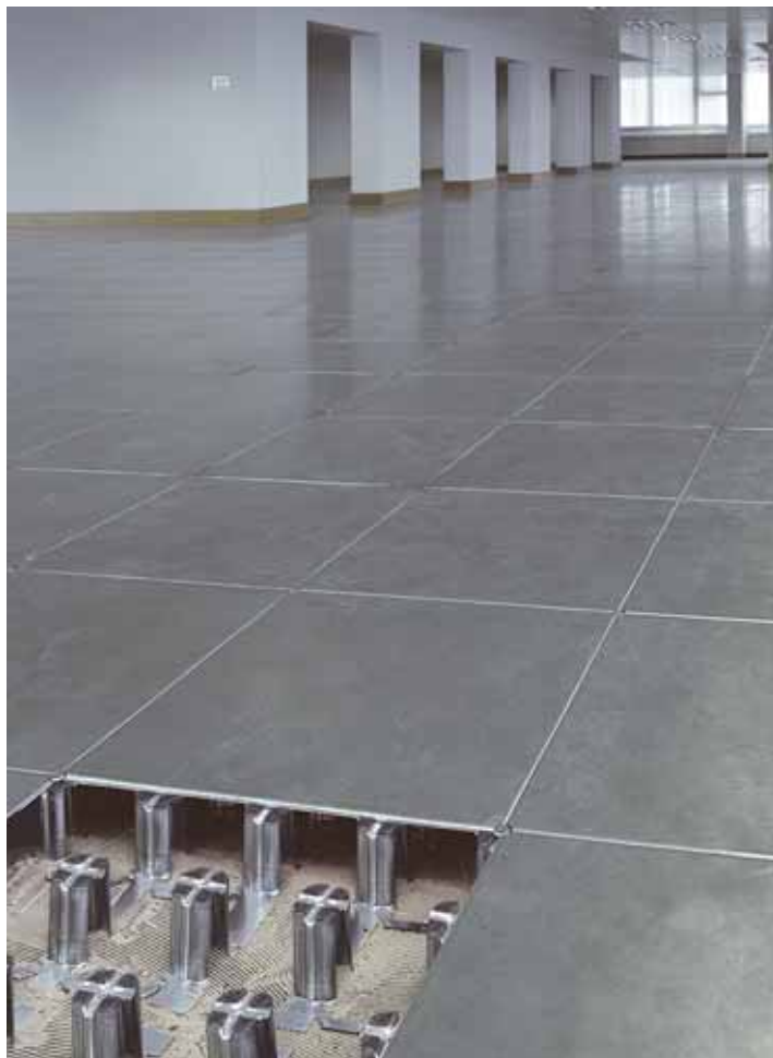
ABOVE: EUSTON TOWER - INTERCELL INSTALLATION
